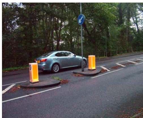
Traffic island adjacent to the school
